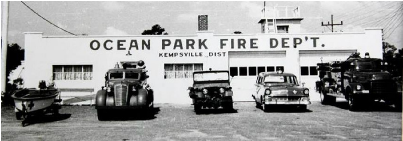
STATION 1 CIRCA 1960. THIS BUILDING SERVES AS THE CURRENT HOME OF OPVRS.
